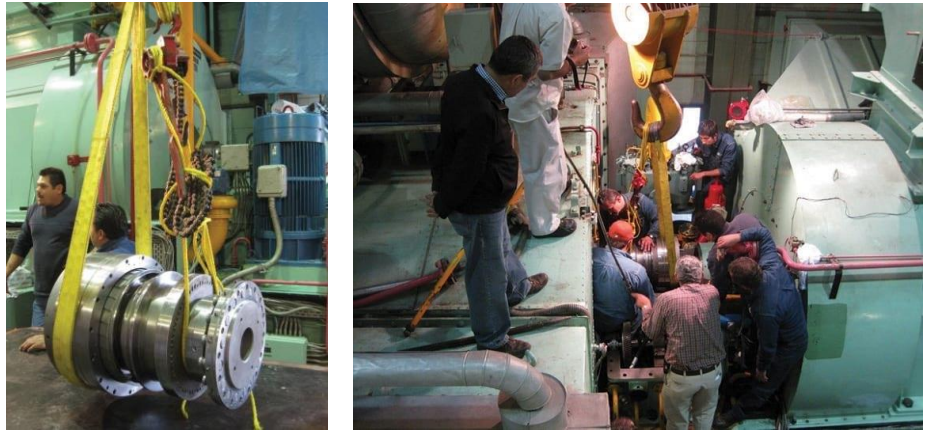
Figure 16: Repurposing of Coal-Fired Steam Turbine into a Synchronous Condenser
